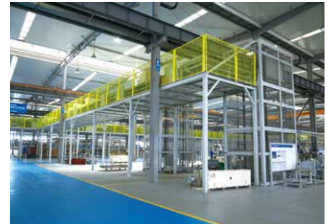
高架物流输送线 Elevated products transport line
